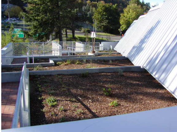
Innovative Stormwater Management, Native American Student and Community Center, Portland State University, Portland, Oregon; Stastny Brun
