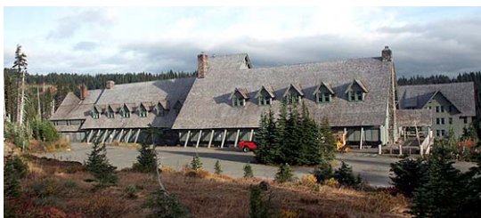
Drainage Improvements, Paradise Inn, Mt. Rainier National Park, Washington; Fletcher Farr Ayotte for the National Park Service
