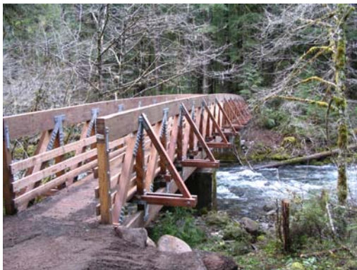
Nohorn Creek Timber Pedestrian Bridge, Bagby Hot Springs, Estacada, Oregon
