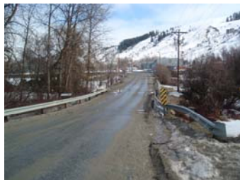
Nespelem School Loop Road and Bridge Improvements, Colville Reservation, Washington
