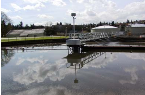
Wastewater Collection and Treatment Facilities Flexible Services Contract, City of Portland, Bureau of Environmental Services
