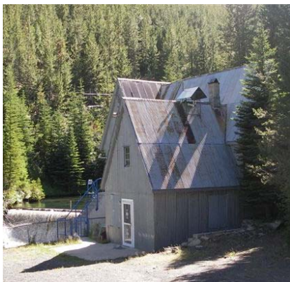
Bend Springs Water Supply Project, Brown & Caldwell for City of Bend, Oregon
